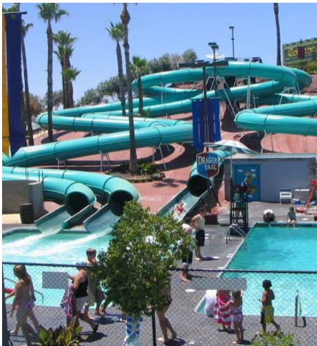
Supported Enclosed Tubular Flume
