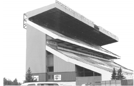
Steel Grandstand – Good Quality (A)
