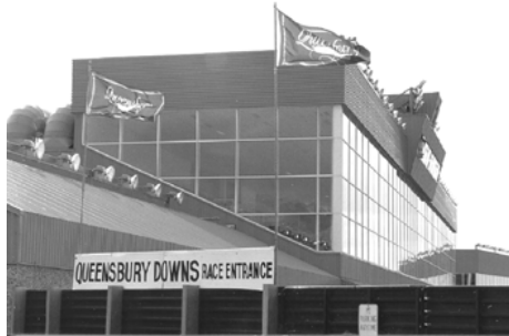
Steel Grandstand – Good Quality (A)
