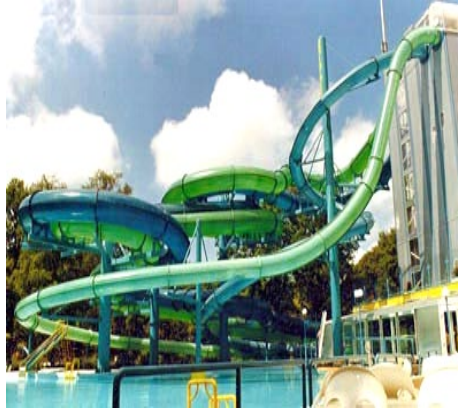
Supported Water Slide
