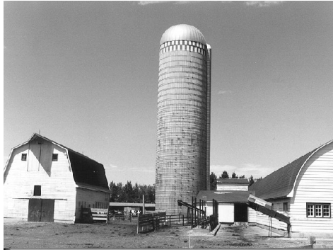
Concrete Poured Silo
