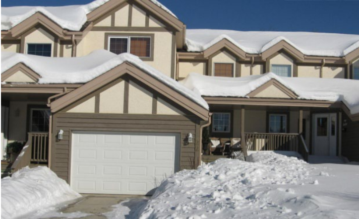
Very Good #1: 2-Storey Townhouse
