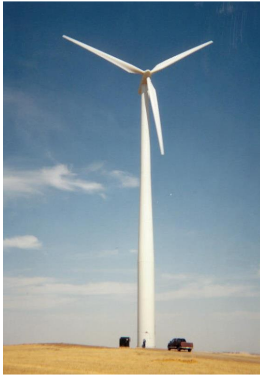
Horizontal Axis Wind Turbine (0.66 MW)
