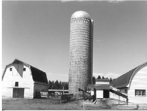
Concrete Poured Silo
