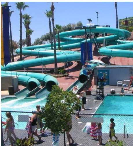
Supported Enclosed Tubular Flume
