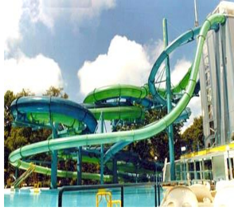
Supported Water Slide
