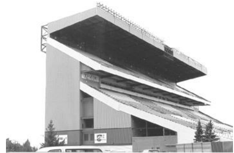
Steel Grandstand – Good Quality (A)
