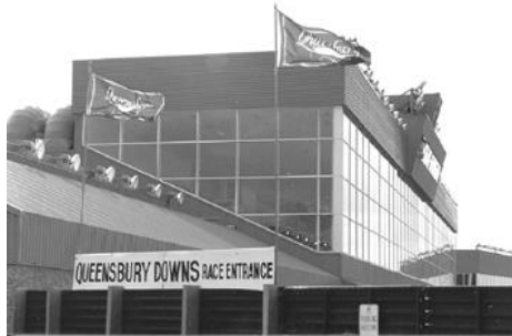
Steel Grandstand – Good Quality (A)
