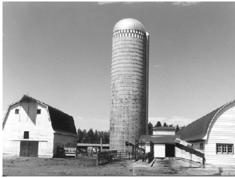
Concrete Poured Silo
