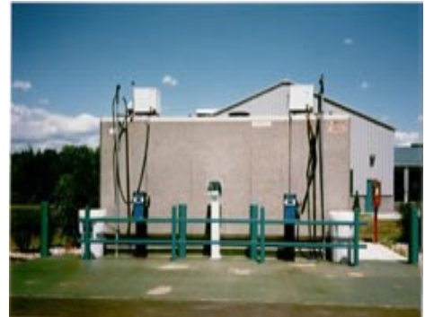
Encased in concrete
